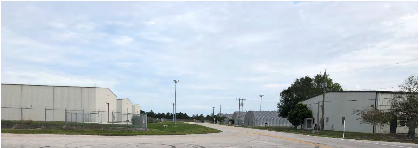
FIGURE 1.35: NORTH RAMP AREA
