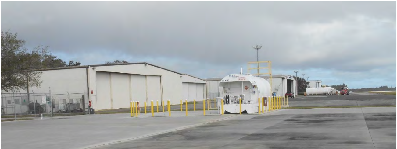
FIGURE 1.34: WEST RAMP LOOKING NORTH
