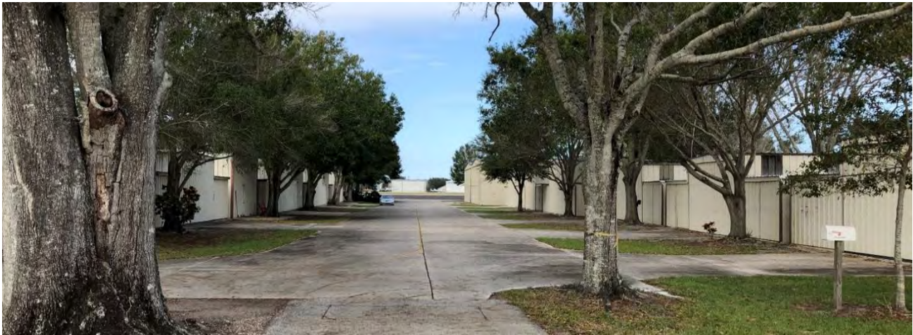
FIGURE 1.33: VRB PORT-A-PORT HANGAR AREA
