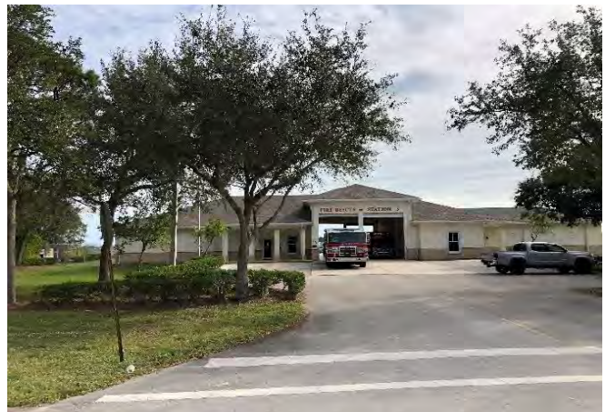
FIGURE 1.52: ARFF STATION (FIRE STATION 3)
