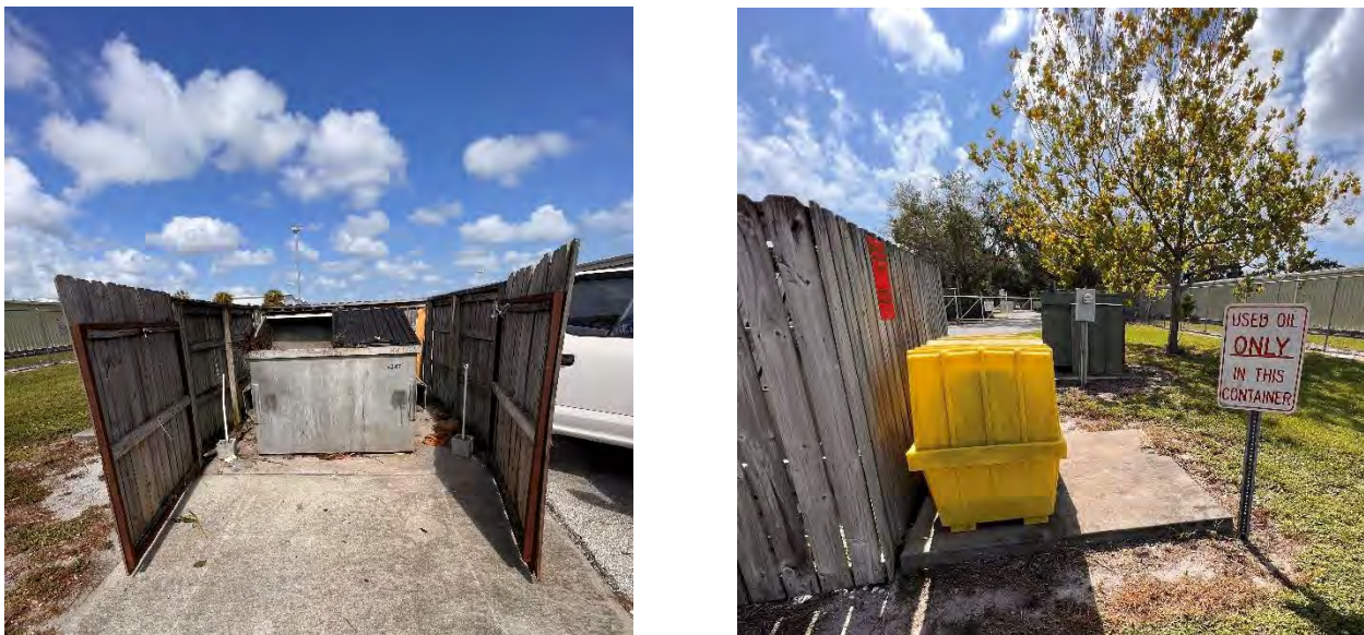
FIGURE 1: DUMPSTER AND WASTE OIL RECEPTACLE IN THE VRB HANGAR AREA
